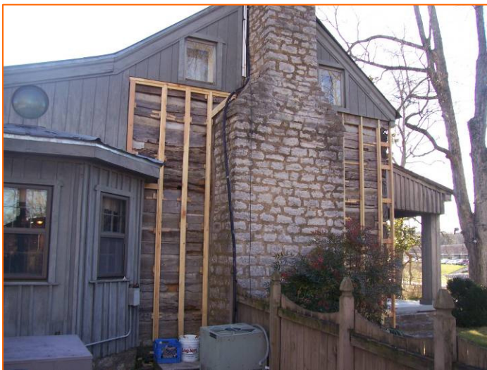
Buchanan Log House west wall and second story repairs. It is believed that the roof leaks are a result of deteriorated logs on the second floor and these repairs should fix those problems. 1-30-2012 Photo by BLH's Joe Cathey
