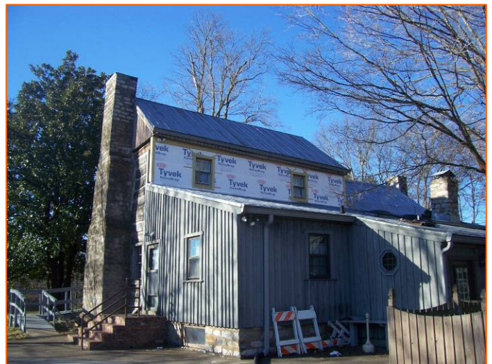
Buchanan Log House west wall and second story repairs. It is believed that the roof leaks are a result of deteriorated logs on the second floor and these repairs should fix those problems. 1-30-2012 Photo by BLH's Joe Cathey
