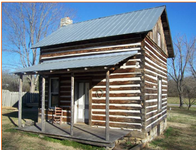
Chinking and log cleaning and preservation have been completed. 1-30-2012 Photo by BLH's Joe Cathey
